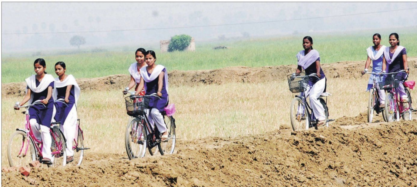
A road under construction in a Bihar village. The states recording highest road construction are Madhya Pradesh (63,548 km), followed by Rajasthan (58,462 km), Uttar Pradesh (45,905 km), Bihar (35,510 km) and Odisha (35,019 km). Prashant Ravi
